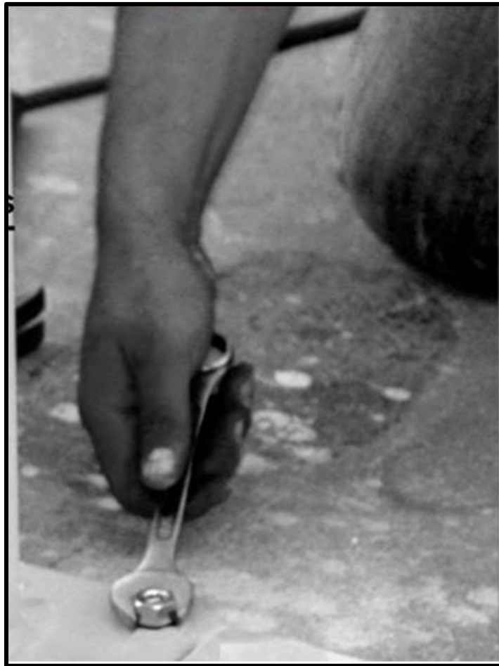
Figure 19 Secure Anchors with Wrench for Final Attachment
