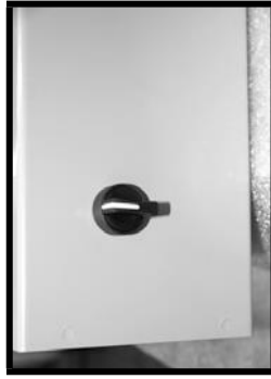
Figure 39 Momentary Switch in OFF or Neutral Position
